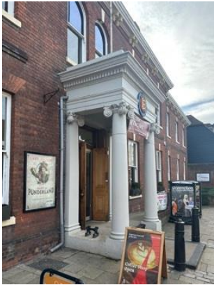
Architectural detail: Building details
