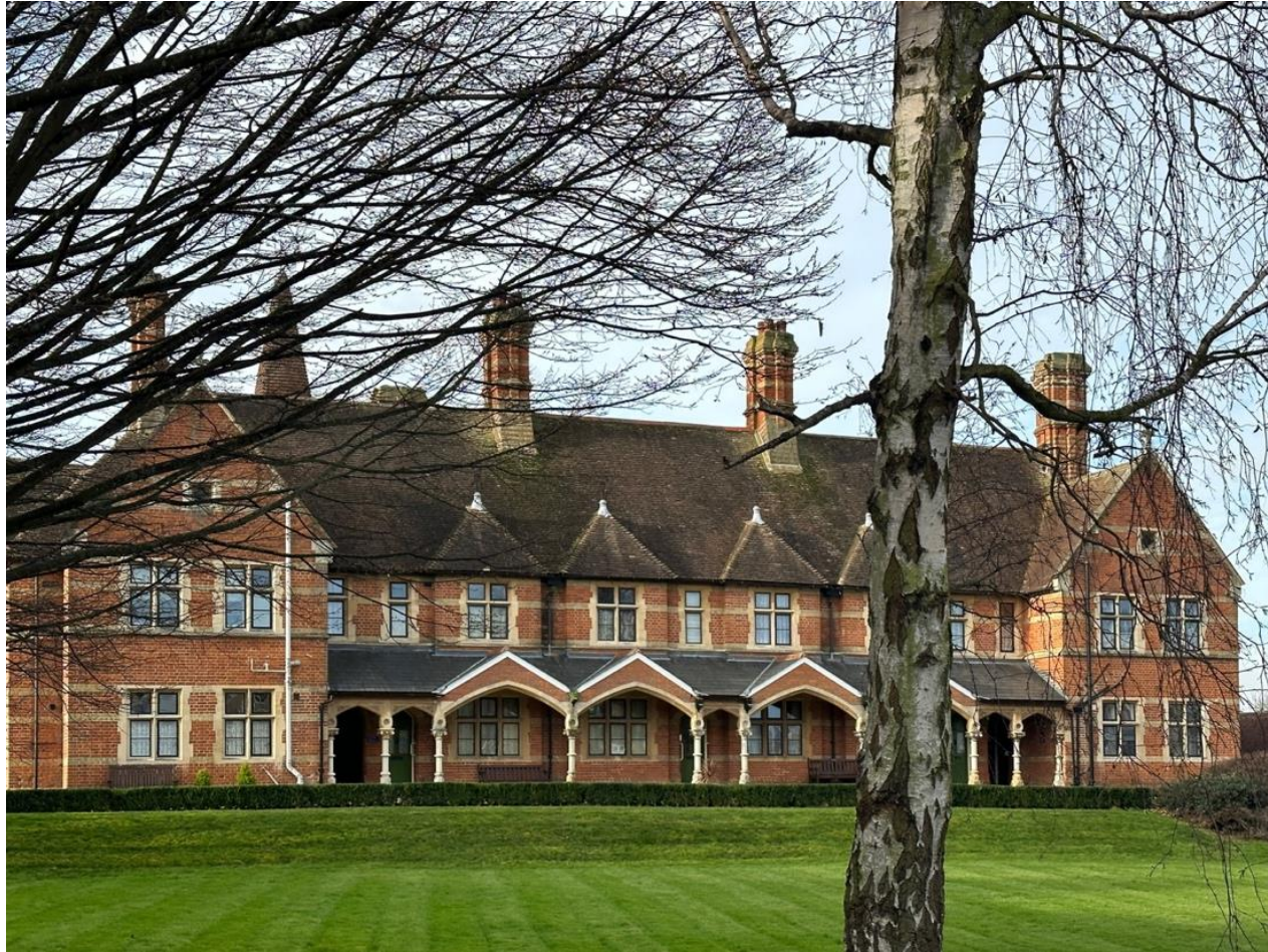
Alms-houses and Chapel 1-30 South Road: listed grade II.
