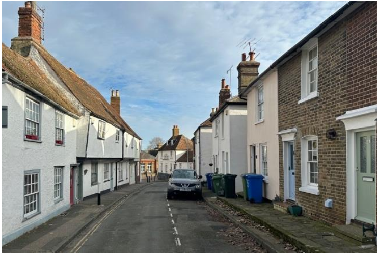
Townscape character in much of the Conservation Area is based on rear of pavement frontages and spaces. This is demonstrated by Tanner Street (left image) and West Street (right image).
