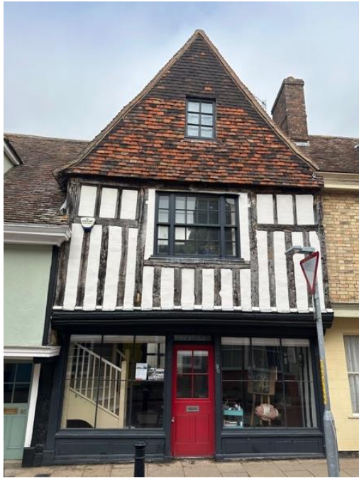
Shopfronts: Traditional historic shopfronts have typical features such as an unusual, curved corner. The jettied (corbelled) form of
